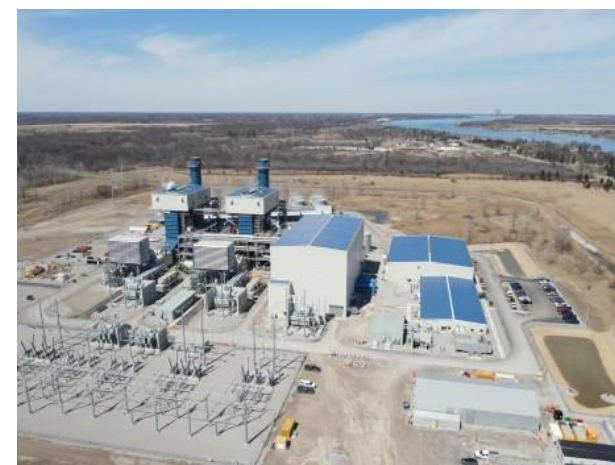
Blue Water Energy Complex NGCC Plant
